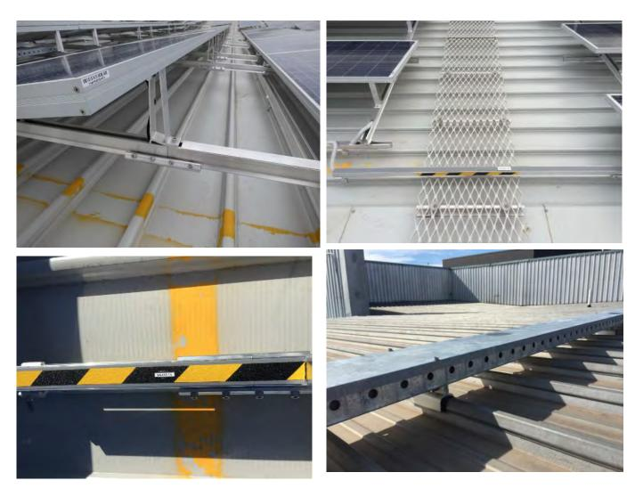
To simplify the installation while achieving best practice, the AC and DC cable trunking was carefully selected to improve the visuals, quality and performance of the system while ensuring mechanical protection.
