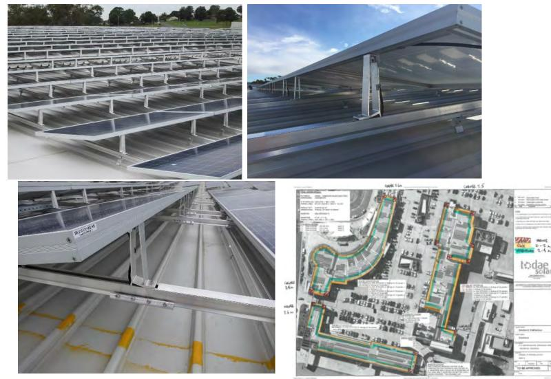
Mount to be structurally adequate and certified for being tilted at 10 degrees with dead load (including panels and other components) to be less than 15kg/m2 and uplift to be less than 2kPa.
