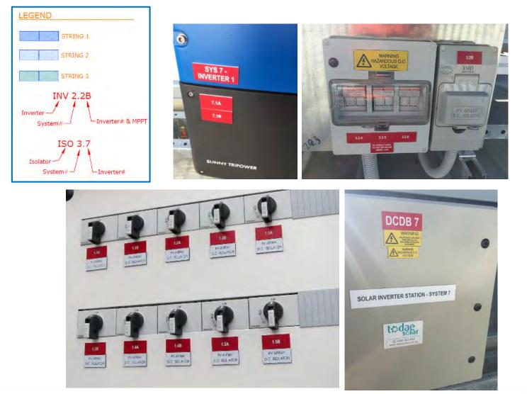
All signage on switches, isolators and within distribution boards and switchboards have to be in accordance with AS 4777 and AS/NZS 5033 and Service and Installation Rules of New South Wales.
